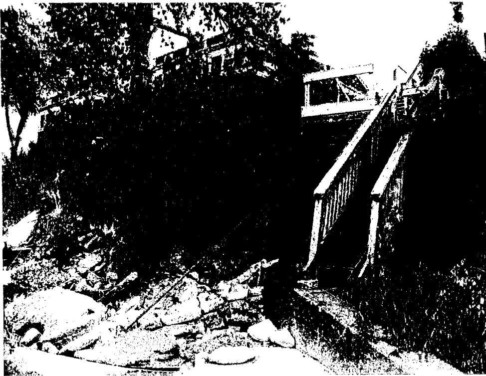
Photo 2: Looking up the bluff from the toe at the west property line.
